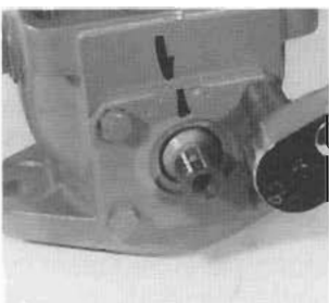
Fig. 26 - Install Trunnion Seal Carrier
